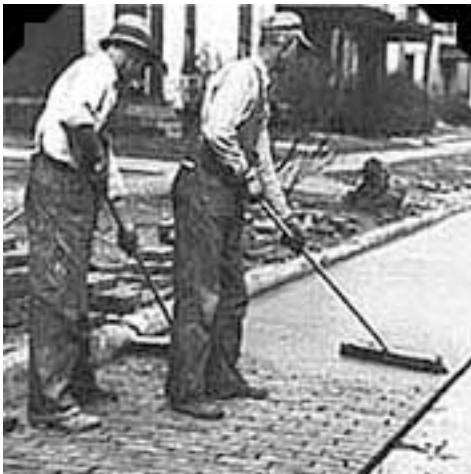
Roadwork accounted by far for the largest number of WPA projects.
