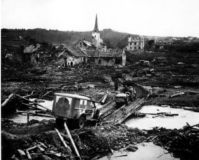
Destruction in Germany, March, 1945
