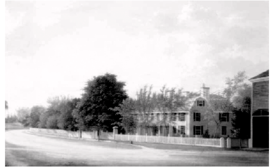
Old House. NATIONAL PARK SERVICE, ADAMS NATIONAL HISTORICAL PARK
