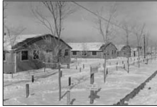
Figure 5.6. Warehouse area at Granada. (Joe McClelland photograph, Bancroft Library, University of California, Berkeley)
