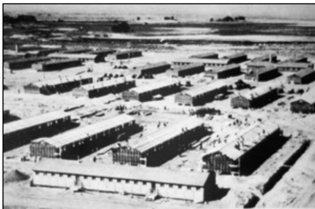
Figure 11.3. Construction underway at the Rohwer Relocation Center.
