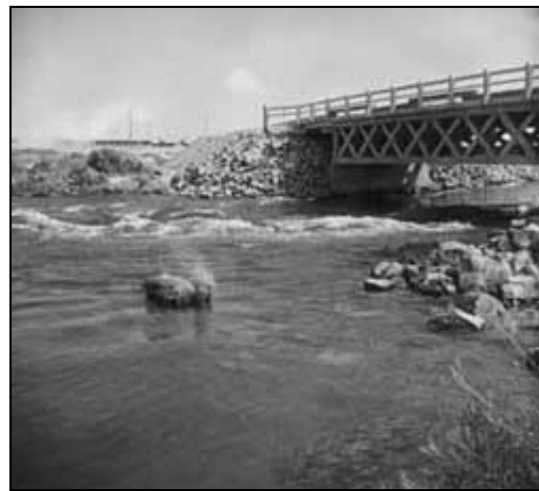
Figure 9.1. North Side Canal.
